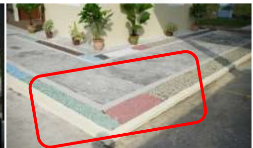
Constructed pavement using plastic aggregates at Geo-polymer House near to UM Bus Station
