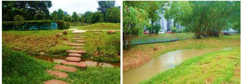
A constructed wetland and stream project at Tasek Varsiti
