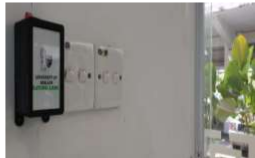
Switch module at Block D, Faculty of Engineering, UM
