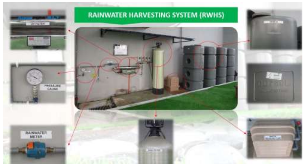
Implementation of Rainwater Harvesting System (RWHS)
