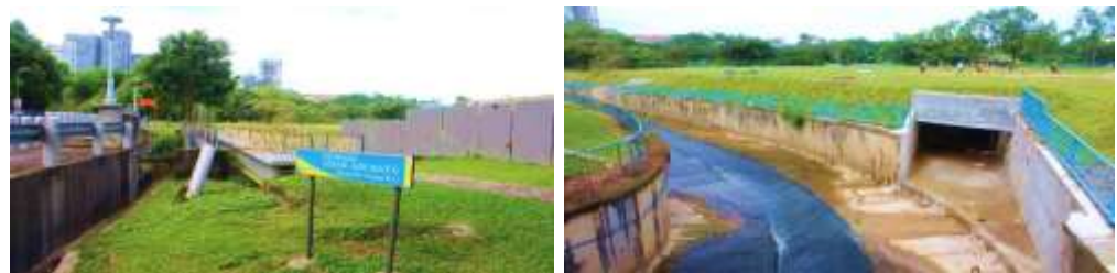
Projek Tebatan Banjir under DBKL: 16,000 metre cube (m3) concealed flood detention pond underground
