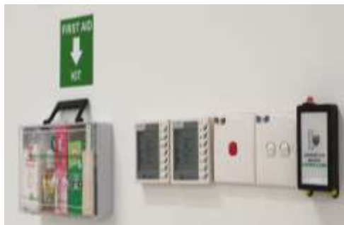
Switch module at Embedded System Lab Block C, Faculty of Engineering, UM
