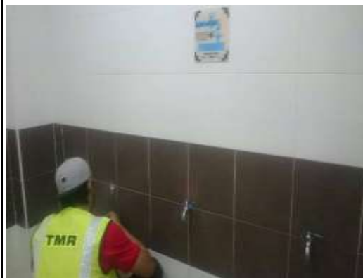
Enhancing the performance of Mr Thimble (low flow device installed from previous phase) at selected musollahs in UM
