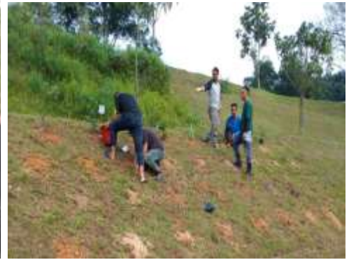
Replanting process of Eco-Slopes
