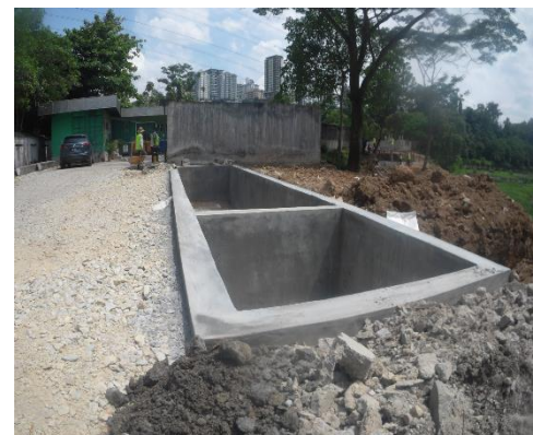
Constructed Wetland project at ZWC to solve leachate problem (JPPHB & OSHE)
