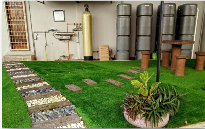
Implementation of Rainwater Harvesting System (RWHS)
