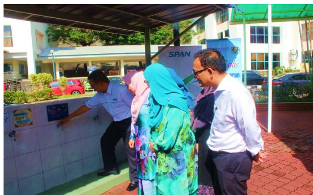
Installation of Cekap Air products in campus
