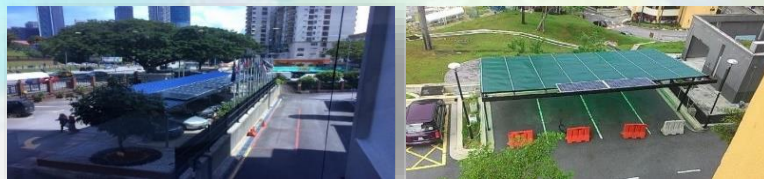
Generating renewable energy through solar panel at rooftop of WISMA R&D parking areas
